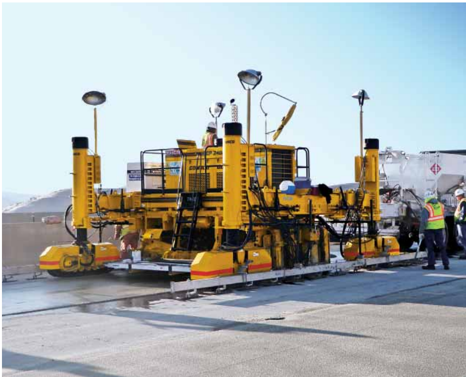
A GP-2400 paves a 0.75 inch (19 mm) thick polymer overlay.
