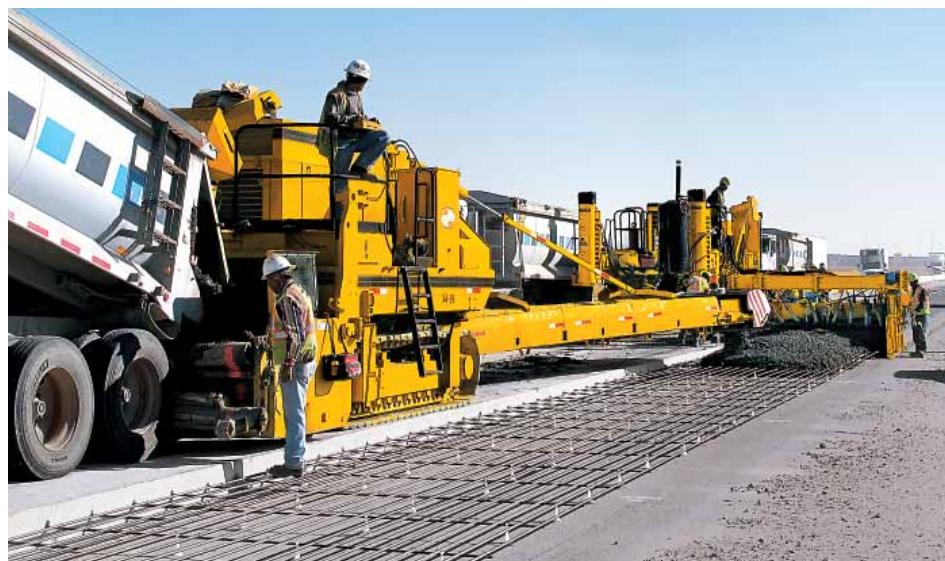
A GOMACO 9500 is placing the concrete over longitudinal steel for the GP-2400 to slipform a scab-on shoulder.
