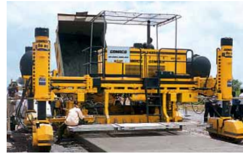
A GP-2400, four-track, paves a new access road for an airport.
