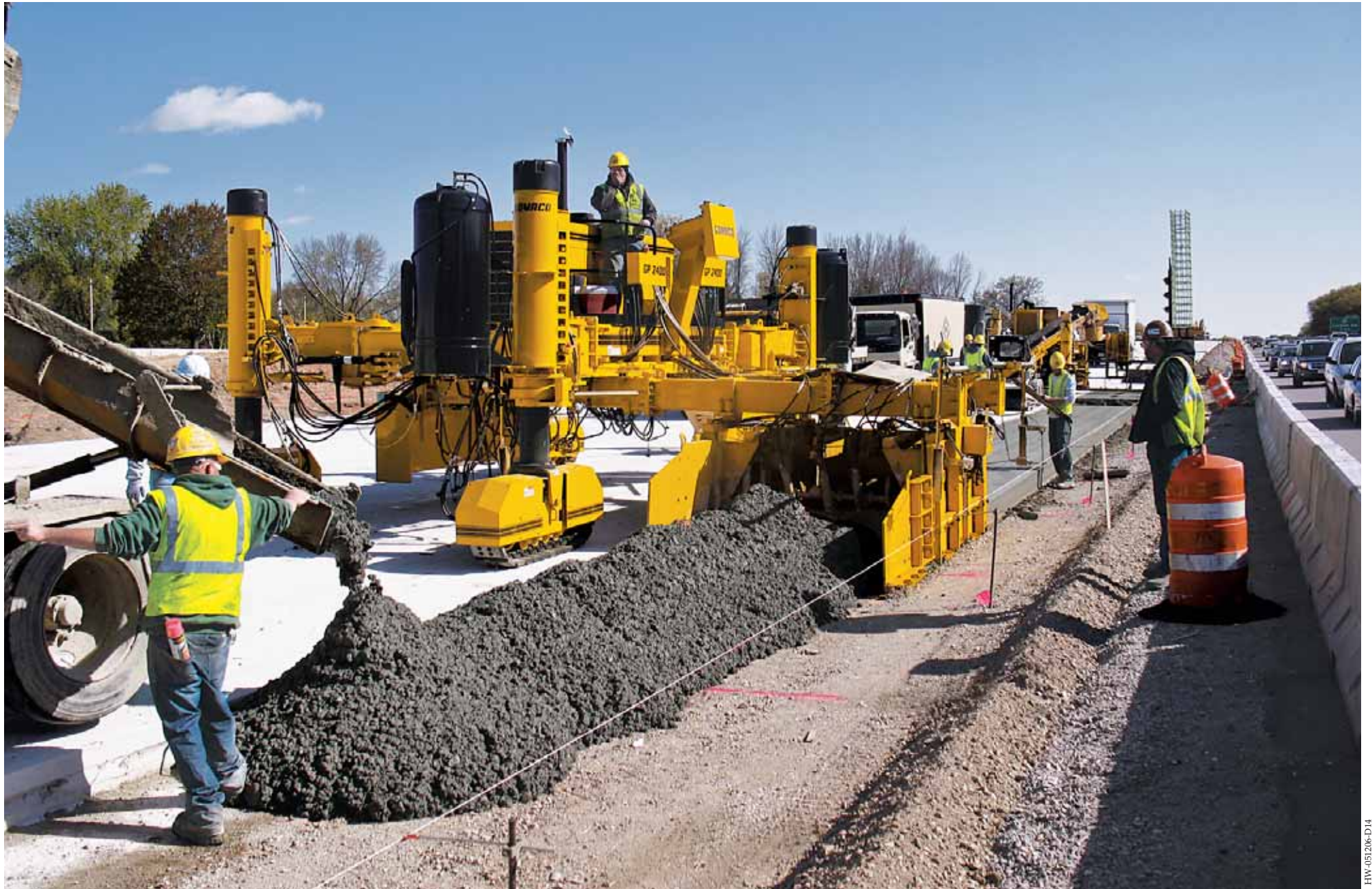
The GP-2400, four-track, paves a 6.5 foot (2 m) wide by 10 inch (254 mm) thick shoulder with a sidemounted mold.
