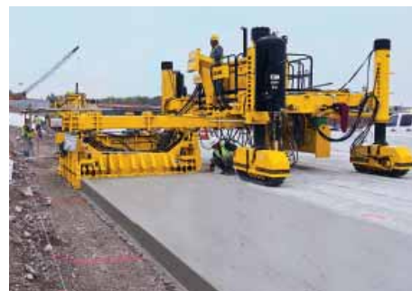
A GP-2400, four-track, paves a 9.25 foot (2.82 m) wide slab that is nine inches (229 mm) thick with a sidemounted mold.
