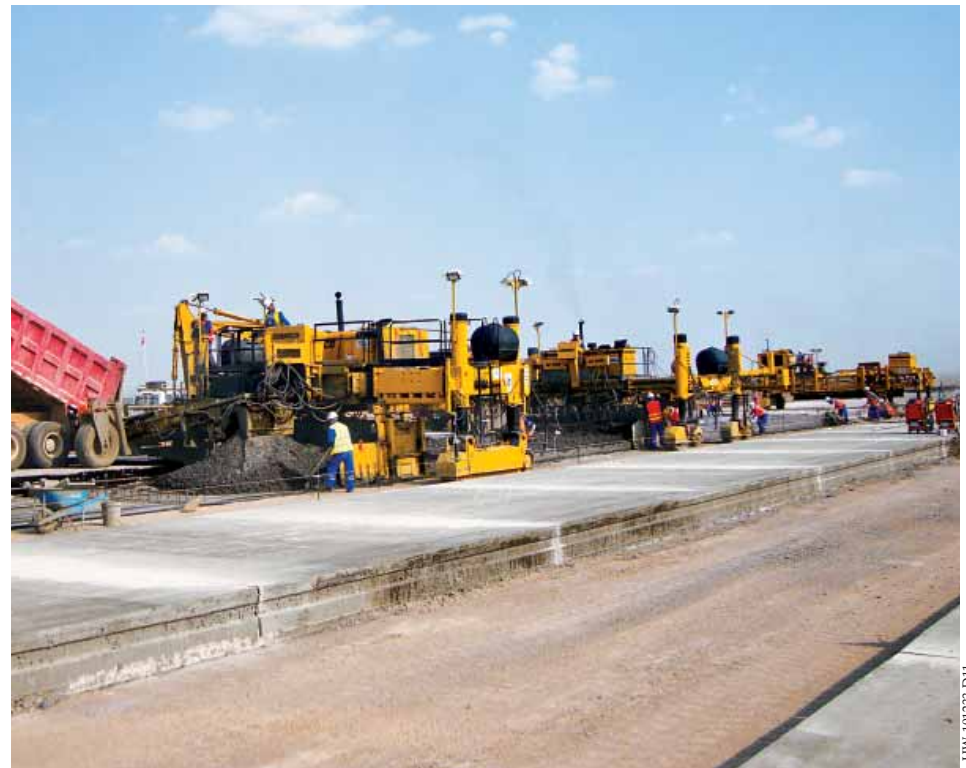
A paving train made up of the PS-2600, GP-2400, and T/C-400 paves an airport strip in a remote area. The airstrip is 10,499 feet (3200.1 m) long.
