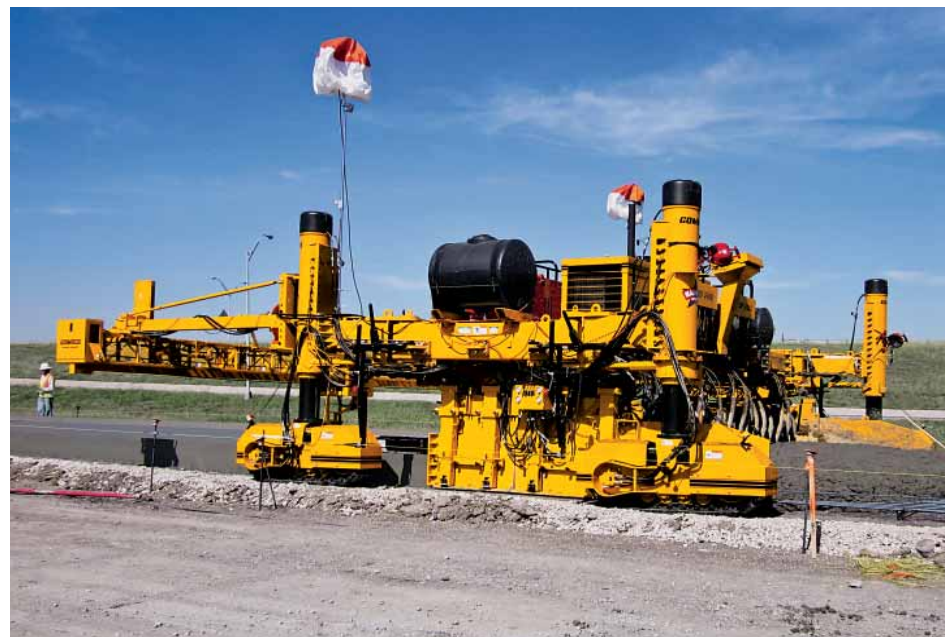
A GP-2400 paves over longitudinal steel and is equipped with the GOMACO Auto-Float®.
