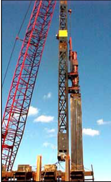
D62-52 in a stand-off driving Kingpile.
